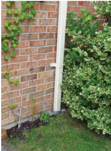
Downspout connected to storm system Kerry Royer, photographer
