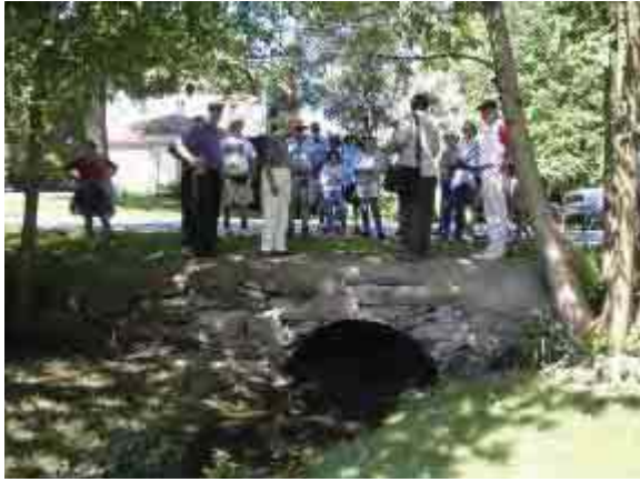
Zone 2 – Undersized Culvert
